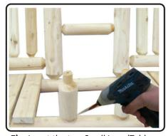
7) Insert the two Small Logs (Table Supports) into the holes between the seats. Insert Screws as shown.
