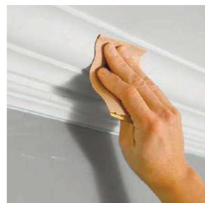
Use sand paper to smooth the surface.
