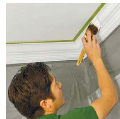
Cover walls and ceiling with tape. Using brush, coat cornice with paint.
