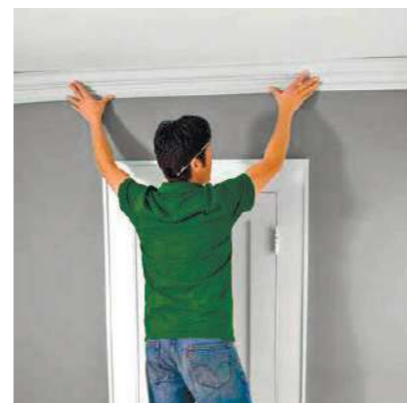
Make markings on the wall using a pencil to define the cornice location
