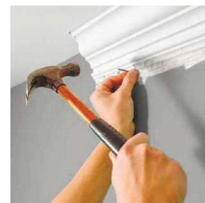
Ensure proper alignment on joints before nailing.
