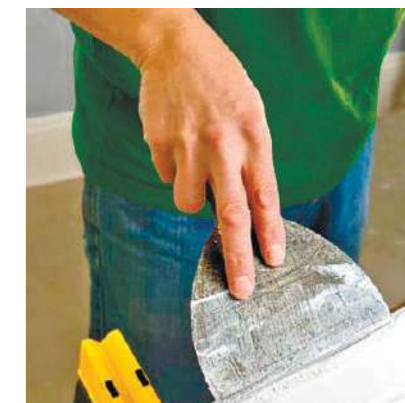
Apply adhesive along the edges at the back of the cornice as well as the mating surface.
